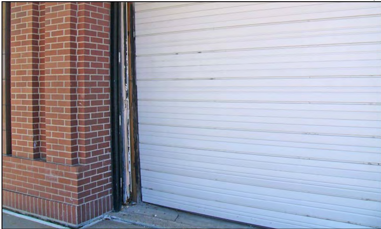
Deteriorated exterior building elements included awnings with peeling paint (above) and cracked or broken frames on windows and doors (below).
