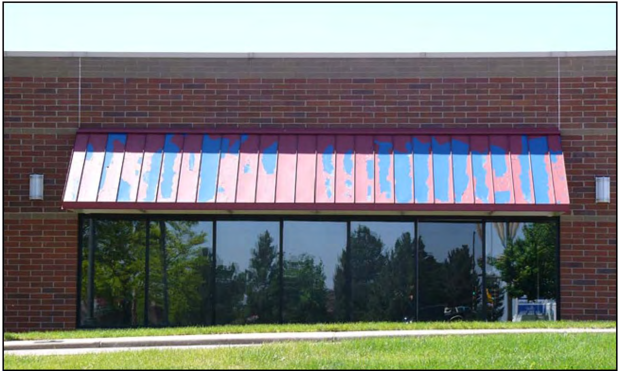
Deteriorated exterior building elements included awnings with peeling paint (above) and cracked or broken frames on windows and doors (below).
