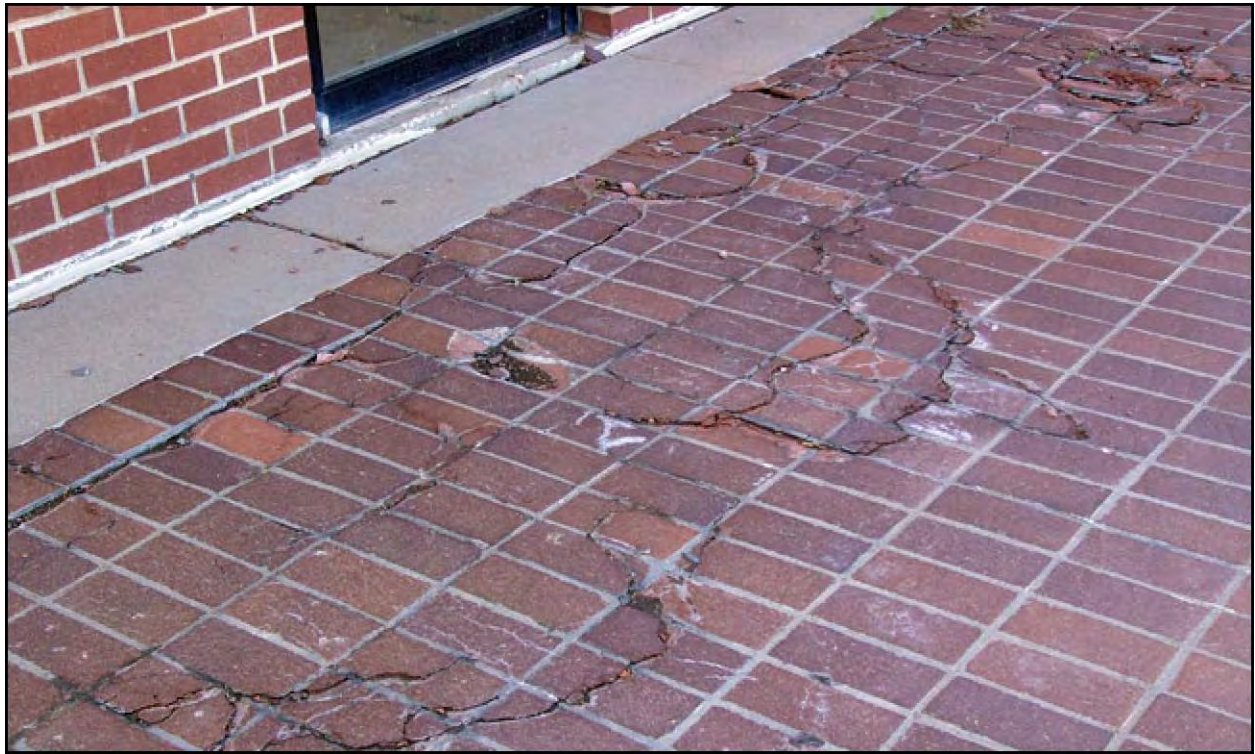
Cracked and buckled sidewalks in retail pedestrian areas and open pot holes in parking areas are examples of unsafe conditions within the Study Area.
